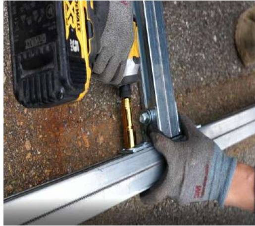
[ Erection of non-welding steel truss ] Assemble segment truss in the factory
