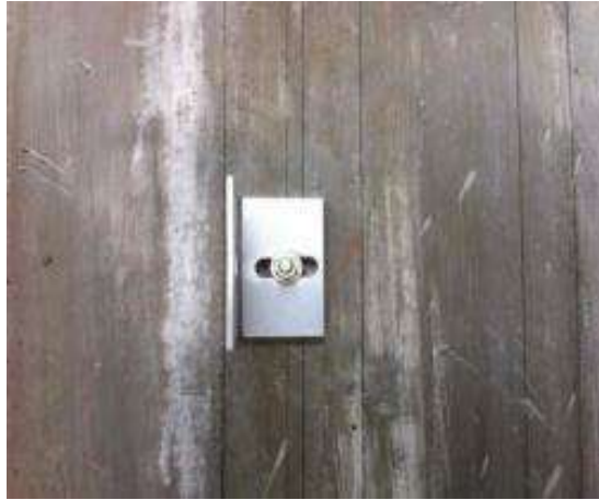
[ Locate fixing bracket ]
