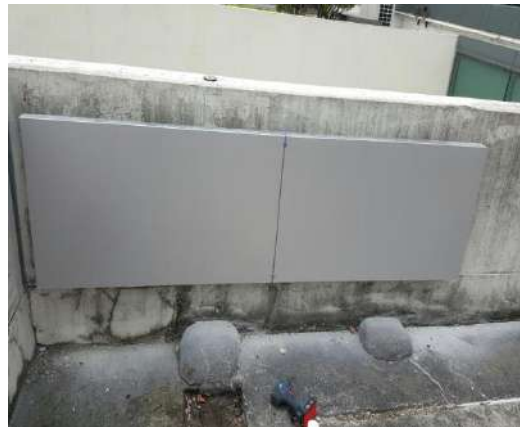
[ Attached Ceramic panel & Curing protection ]
