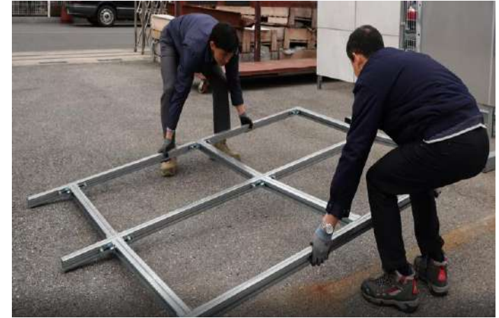
[ Erection of non-welding steel truss ] Assemble segment truss in the factory
