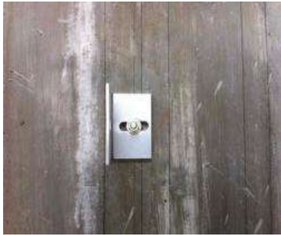
[ Locate fixing bracket ]
