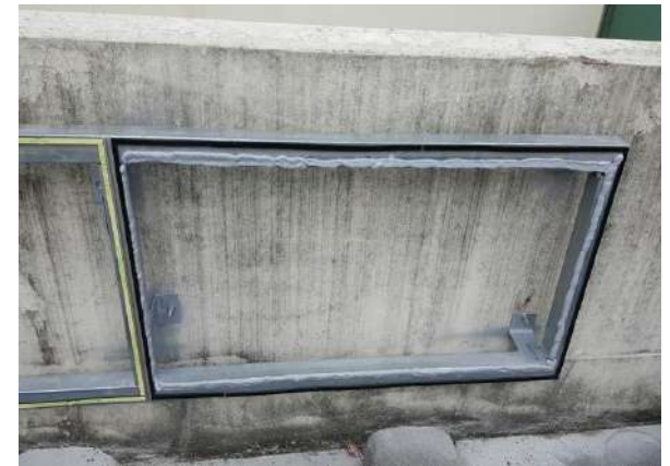
[ Apply Structural sealant ]
