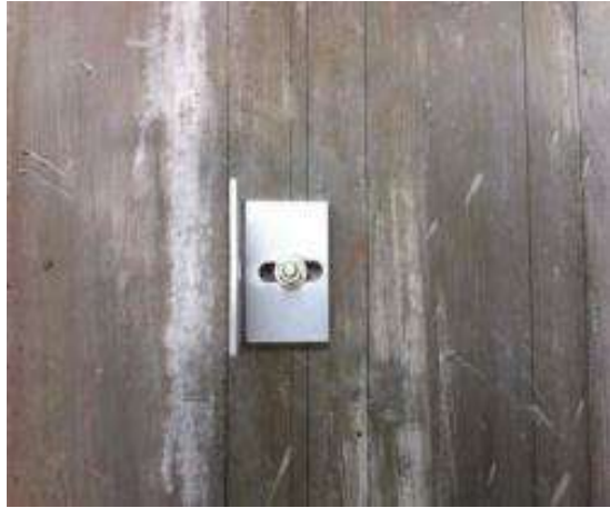
[ Locate fixing bracket ]
