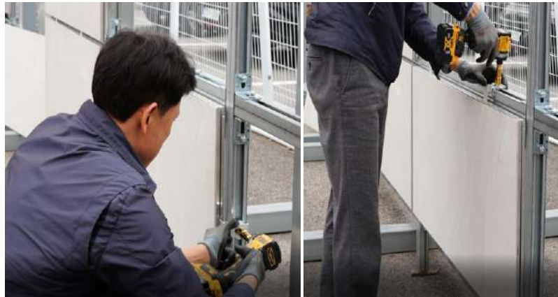
[ Fixing ceramic molding panel ] By Clip
